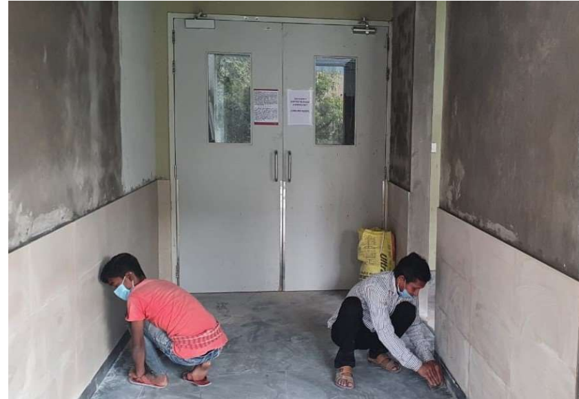
Tata Medical Center Operation Theatre - Construction
