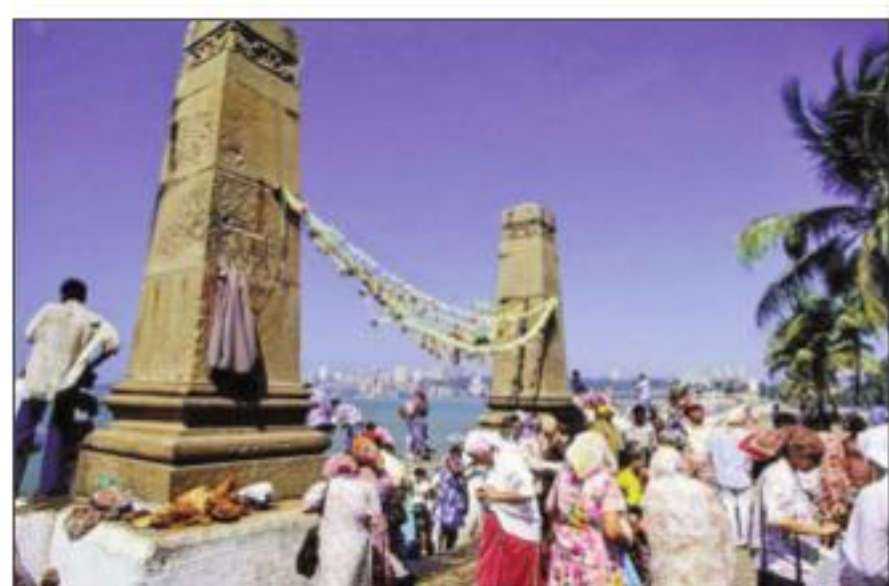
According to the alternative design submitted by the Parsi community, the proposed tunnel could be constructed in the middle of the road instead of building it on the outer edges. This way it would also not affect the century-old Parsi Gate at Marine Drive
