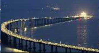
Hong Kong-Zhuhai-Macau Bridge
