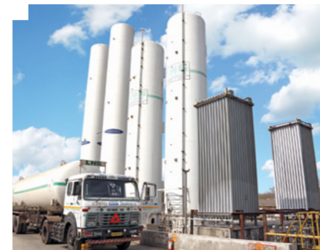
IndianOil, through its Joint Venture Company, IndianOil LNG Pvt. Ltd., has developed a 5-million metric tonnes per annum (MMTPA) capacity Liquefied Natural Gas (LNG) Terminal at Kamarajar Port, Ennore in Tamil Nadu
