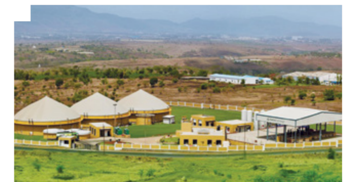
IndianOil's CBG Plant in Pune
