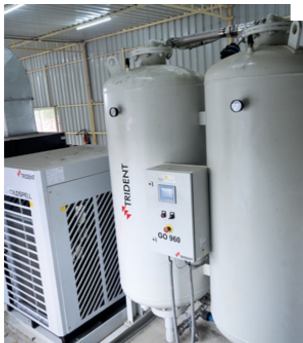
In the backdrop of an acute oxygen availability crisis in the country during Covid-19 pandemic, IndianOil set up Pressure Swing Adsorption (PSA) medical oxygen generation plants at different locations
