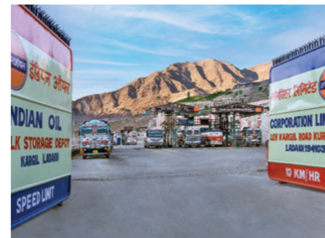
IndianOil's highest altitude bulk storage depot at Kargil
