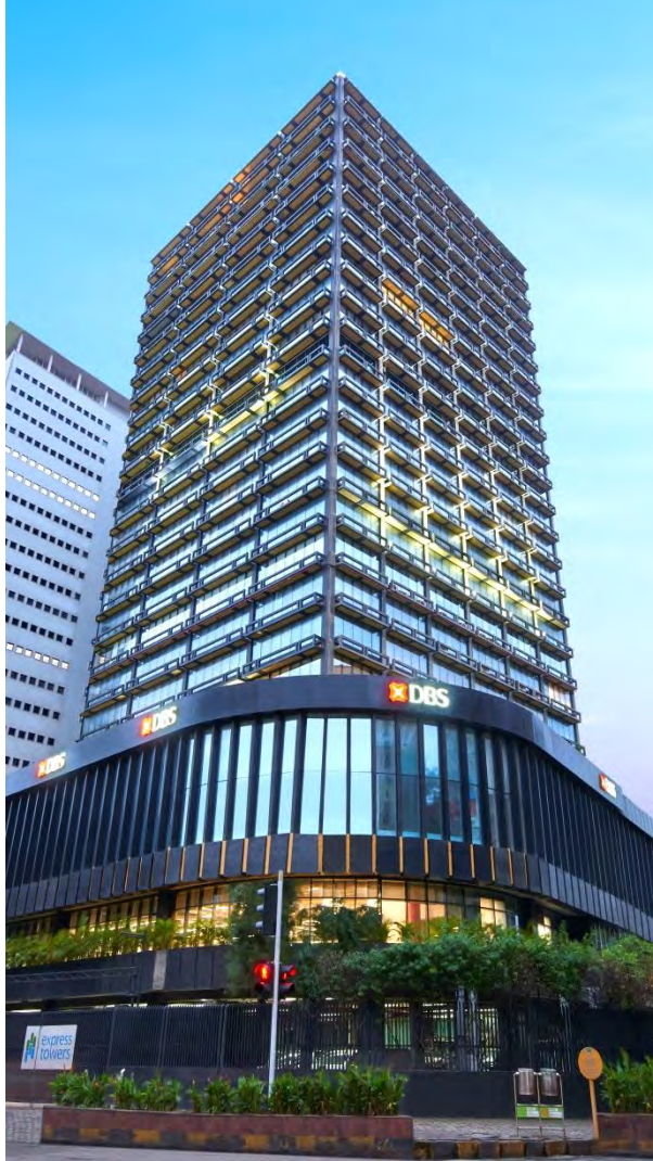
Express Towers Mumbai (0.5 msf)
