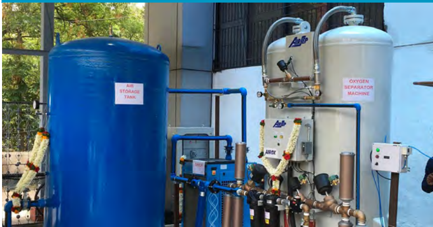
On-site Medical Oxygen Plant (supporting 209 hospital beds)
