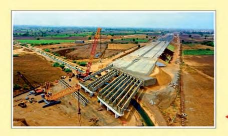
2x400 MT crawler crane deployed for National Highway project in Gujarat for erection of 80 MT girders.
