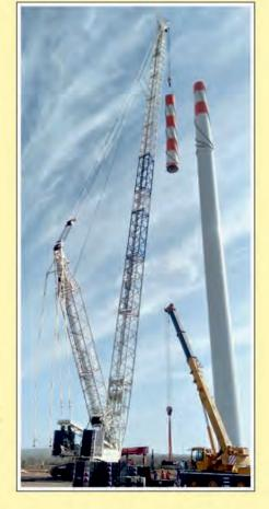
600 MT crawler crane utilized for the erection of a WTG of 130 m hub height in Gujarat.
