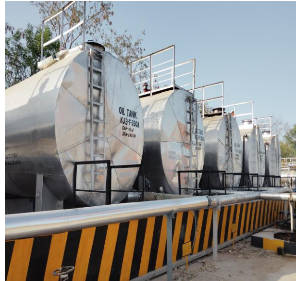
Karjisan Surface Facility Oil storage area
