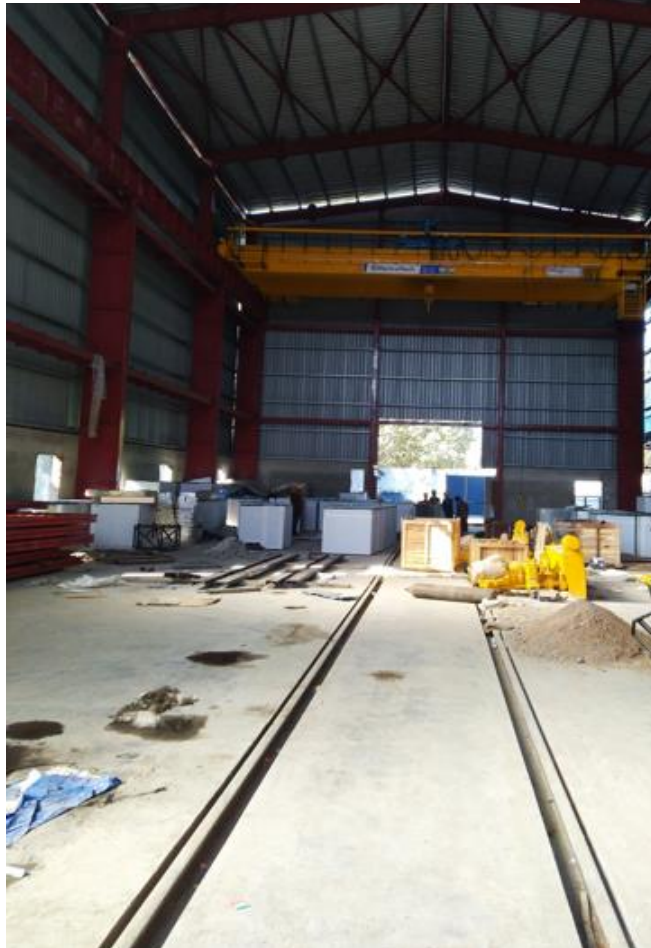
Clean room Shed Odhav
