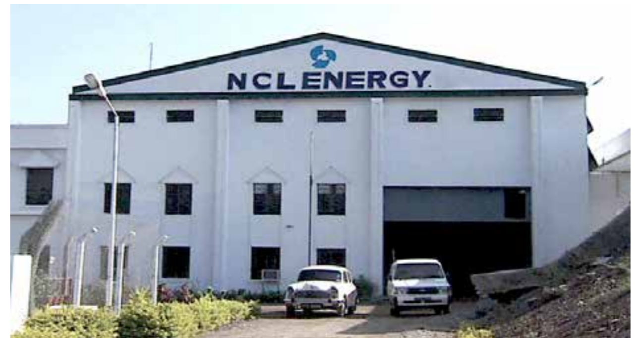
Hydel Power House at Sri Sailam Dam
