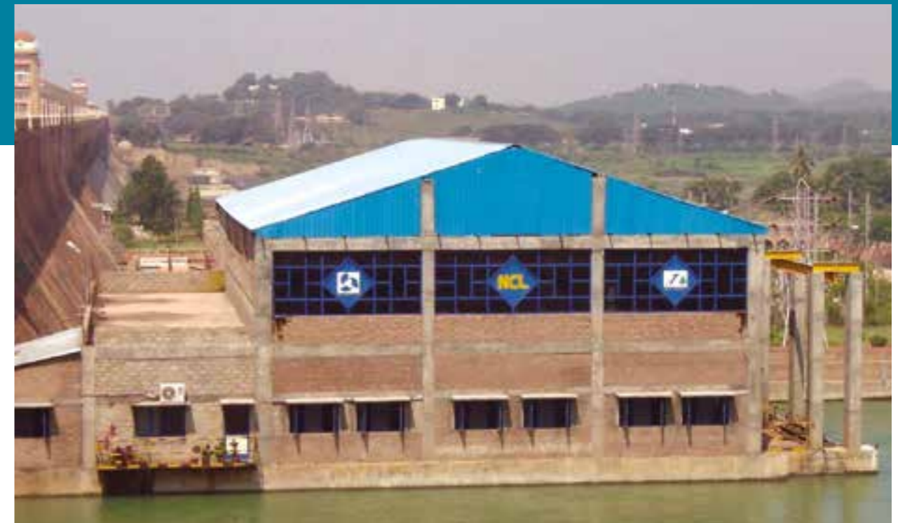
Hydel Power House at Tungabhadra Dam.
