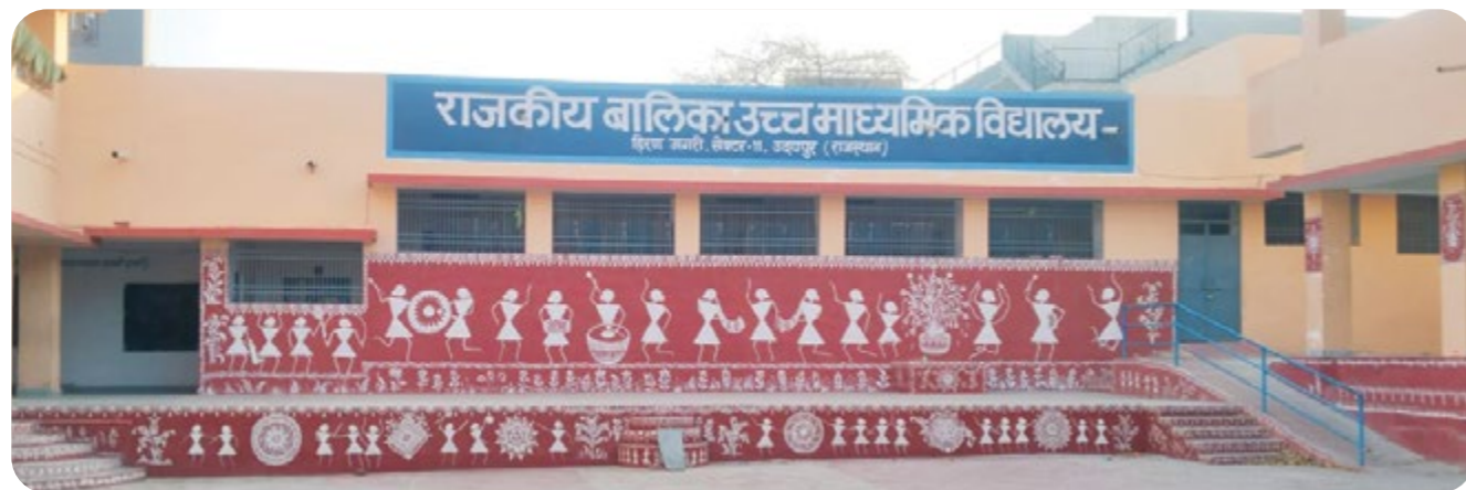
Construction of classrooms at Government Girls Sr. Sec. School, Udaipur, Rajasthan
