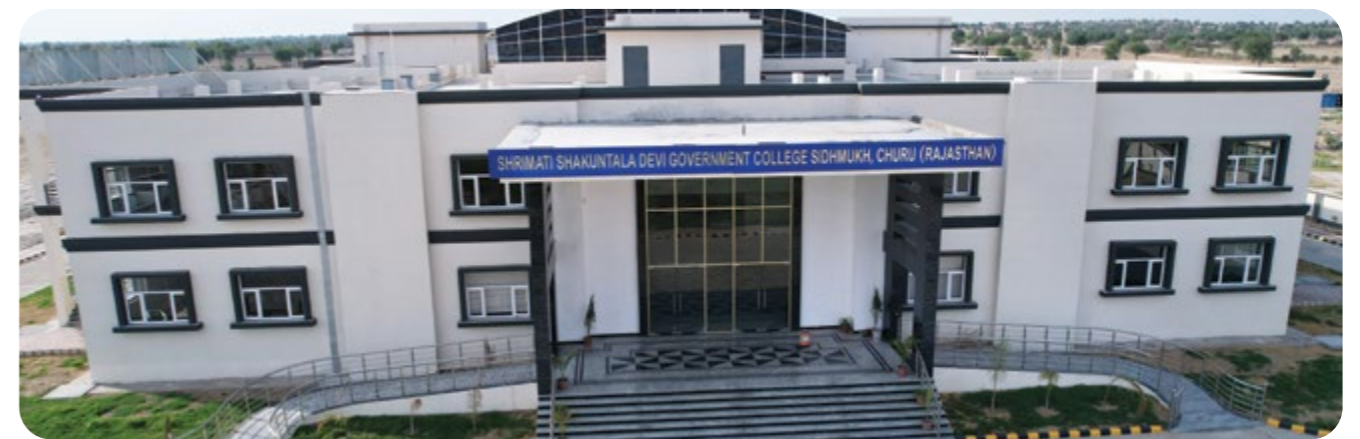
Construction of Smt. Shakuntala Devi Government College Sidhmukh, Churu, Rajasthan
