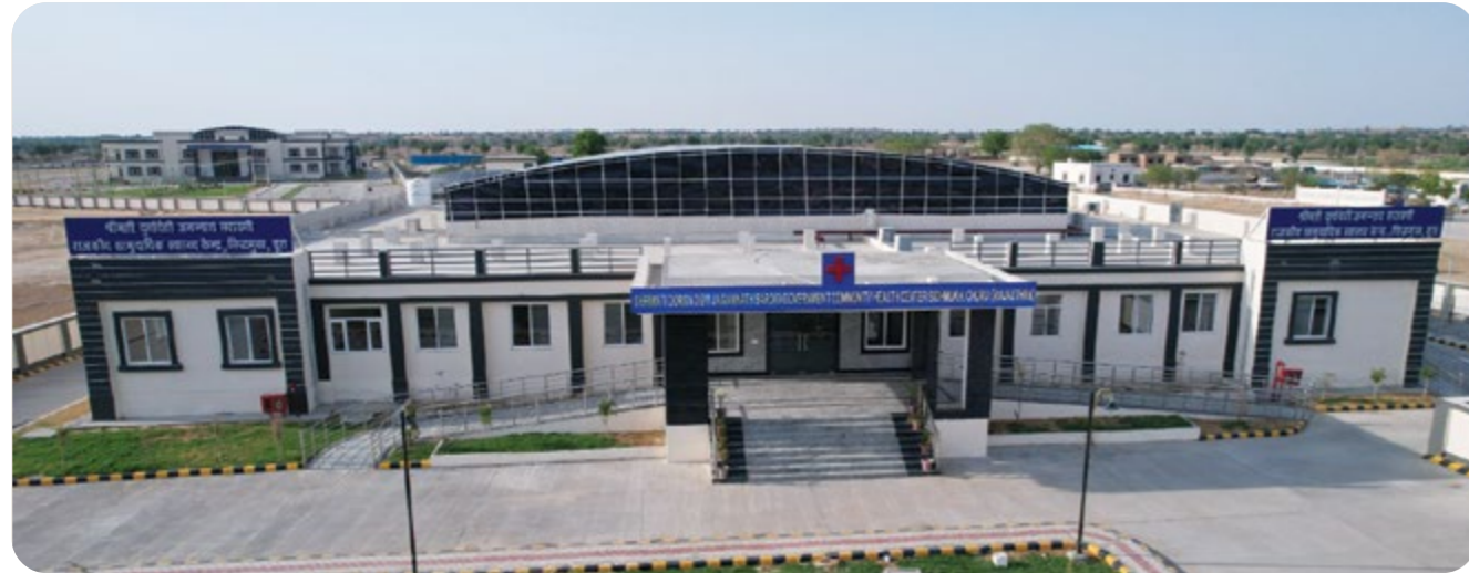
Construction of Smt. Durga Devi Jagannath Sarogi Government Community Health Center, Sidhmukh, Churu, Rajasthan
