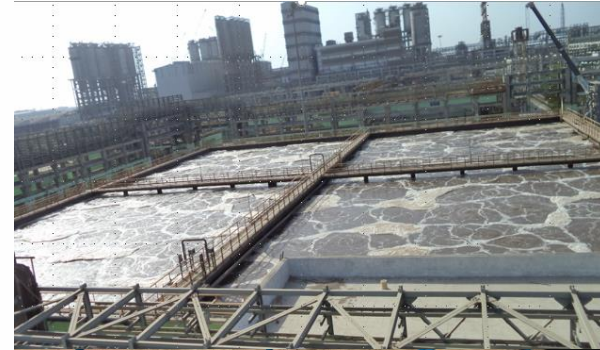
Highly Commended Award under "Industrial project of the Year" for our Dahej Effluent Treatment Plant, India
