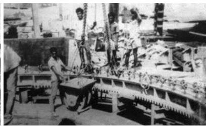
Erection of Bath Rotation Wheel
