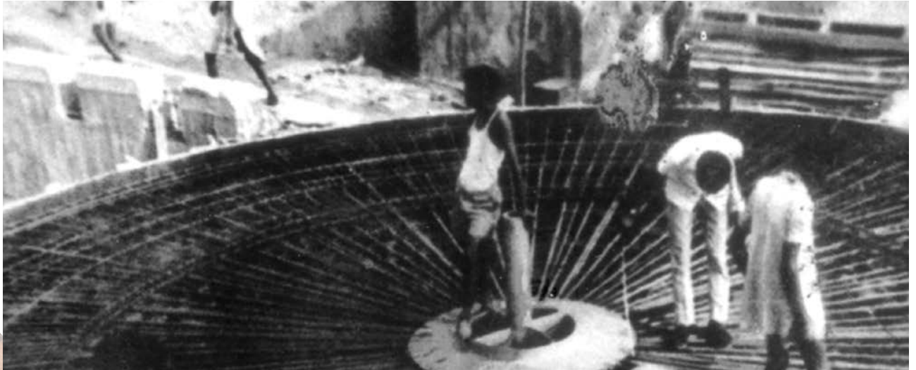
Erection of Furnace Bottom
