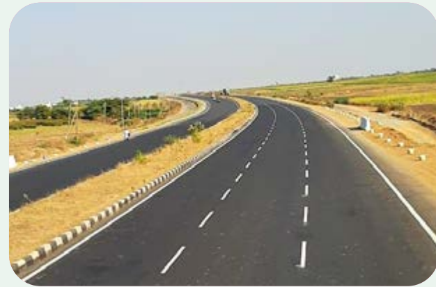
Road markings by AP-PPG
