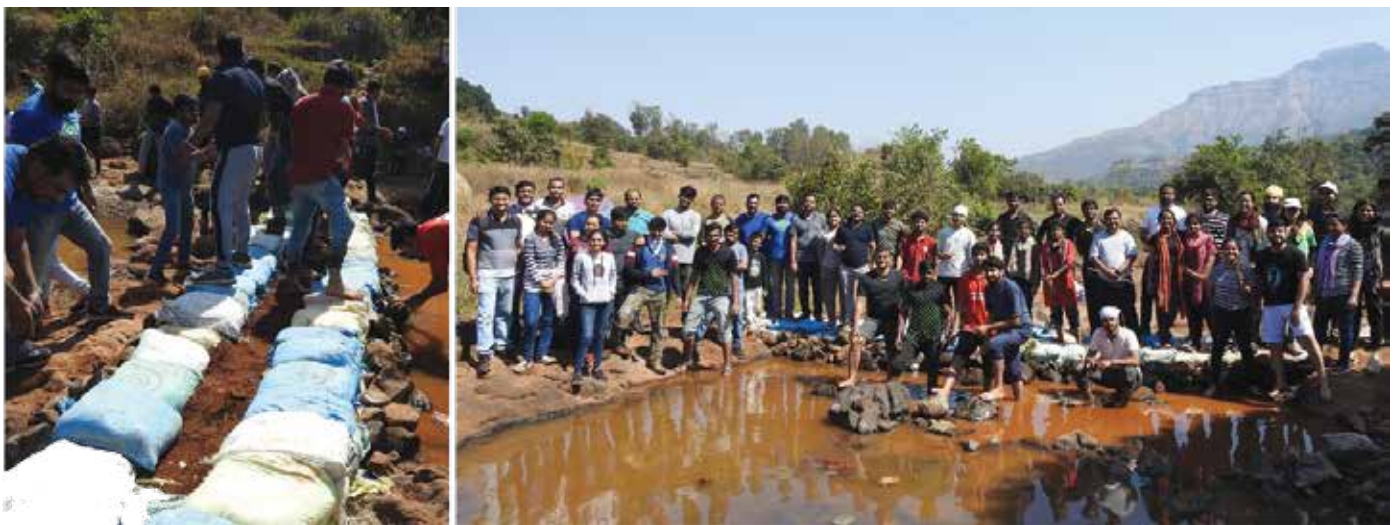
Figure 10: Enthusiastic KPITians constructing the Vanrai Dam
