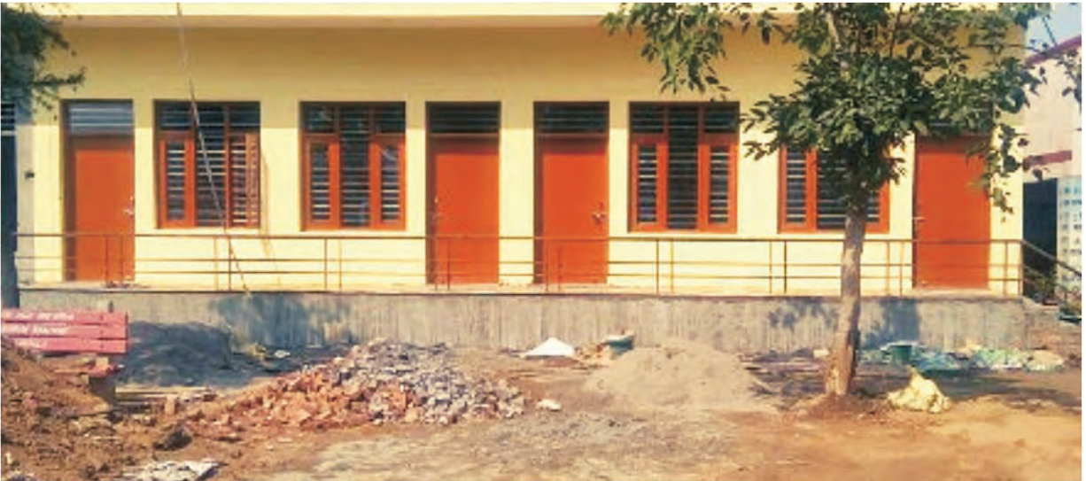
The Company constructed 2 rooms at Tehri School, Patiala.
