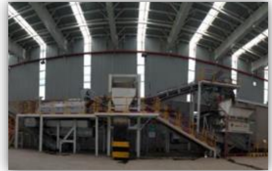
State of art waste processing facility
