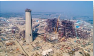
2X660 MW at Rampal, Maitree, Bangladesh-BIFPCL
