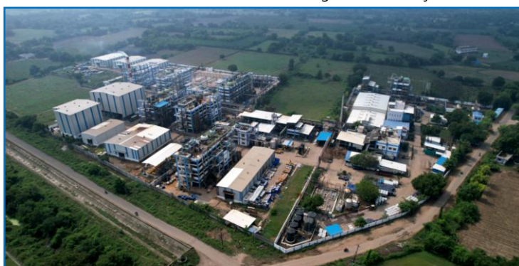
Manufacturing Plants at Manjusar, Vadodara
