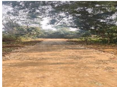
Approach road to wellsite
