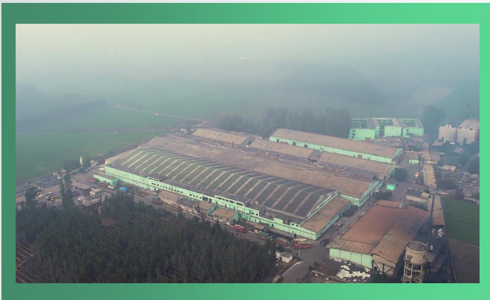
Drone Picture of Shiva Textfab Ltd. based in Ludhiana, Punjab, 100-acre state-of-the-art facility proudly stands as India's preeminent integrated manufacturing unit for rPET waste recycling
