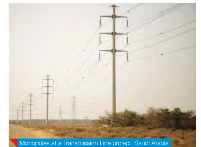
Monopoles at a Transmission Line project, Saudi Arabia
