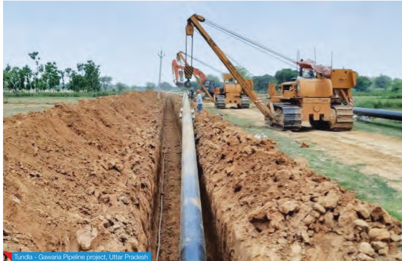
Tundla - Gawaria Pipeline project, Uttar Pradesh
