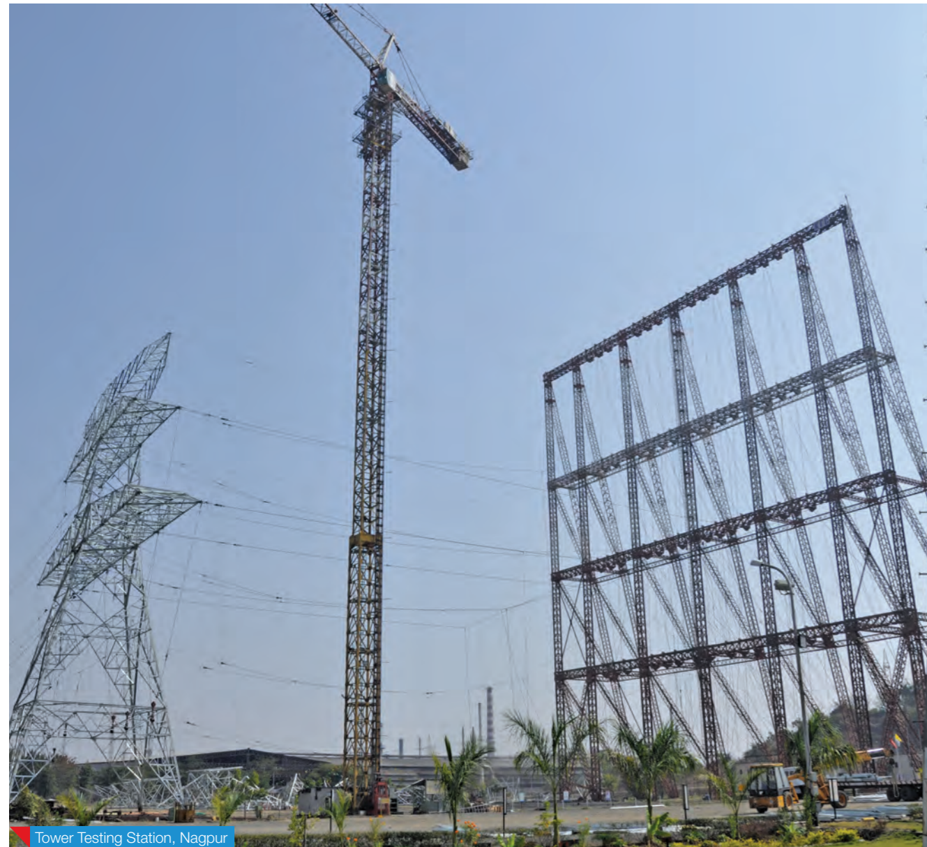
Tower Testing Station, Nagpur
