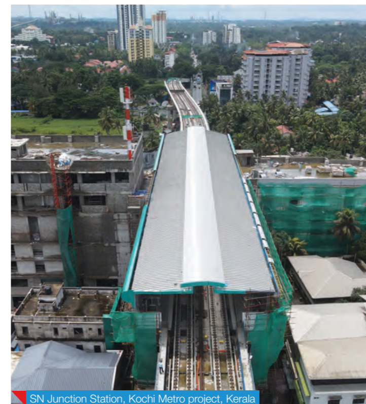
SN Junction Station, Kochi Metro project, Kerala
