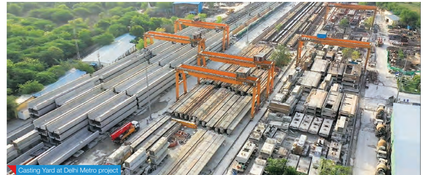
Casting Yard at Delhi Metro project
