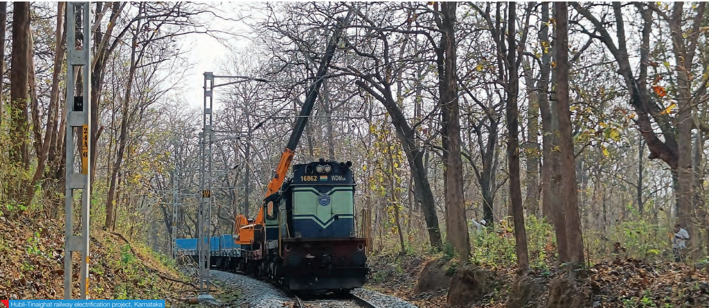
Hubli-Tinaighat railway electrification project, Karnataka
