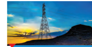
400 kV Overhead Transmission Line project, Saudi Arabia
