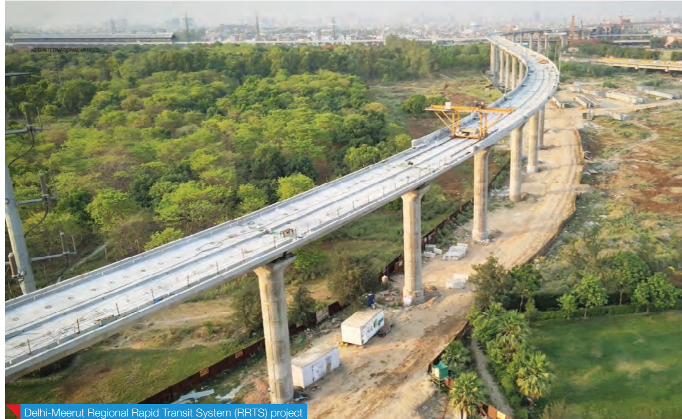
Delhi-Meerut Regional Rapid Transit System (RRTS) project
