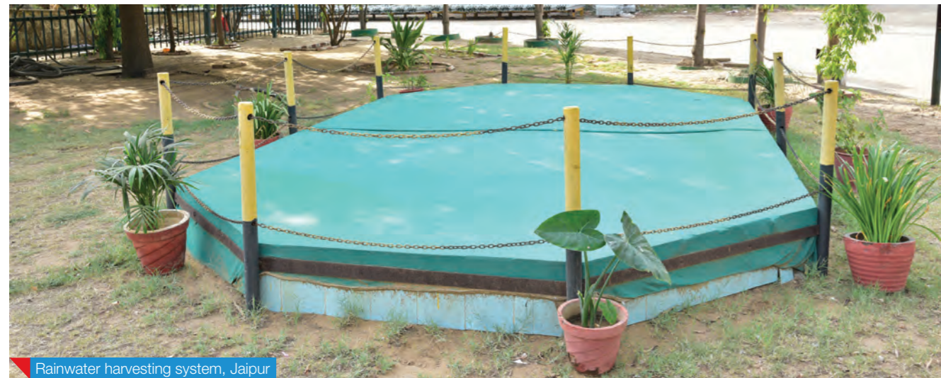
Rainwater harvesting system, Jaipur
