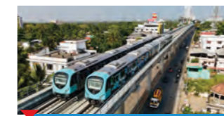
Viaduct and Ballastless Tracks, Kochi Metro Rail Project, Kerala
