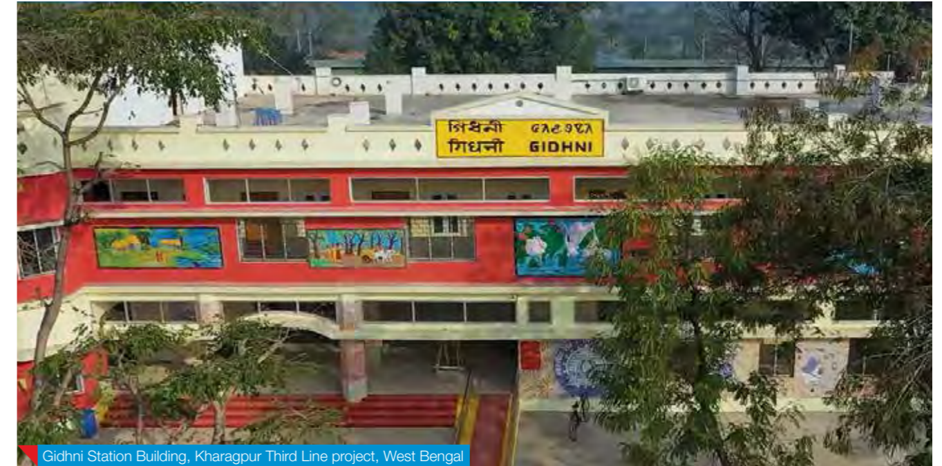
Gidhni Station Building, Kharagpur Third Line project, West Bengal
