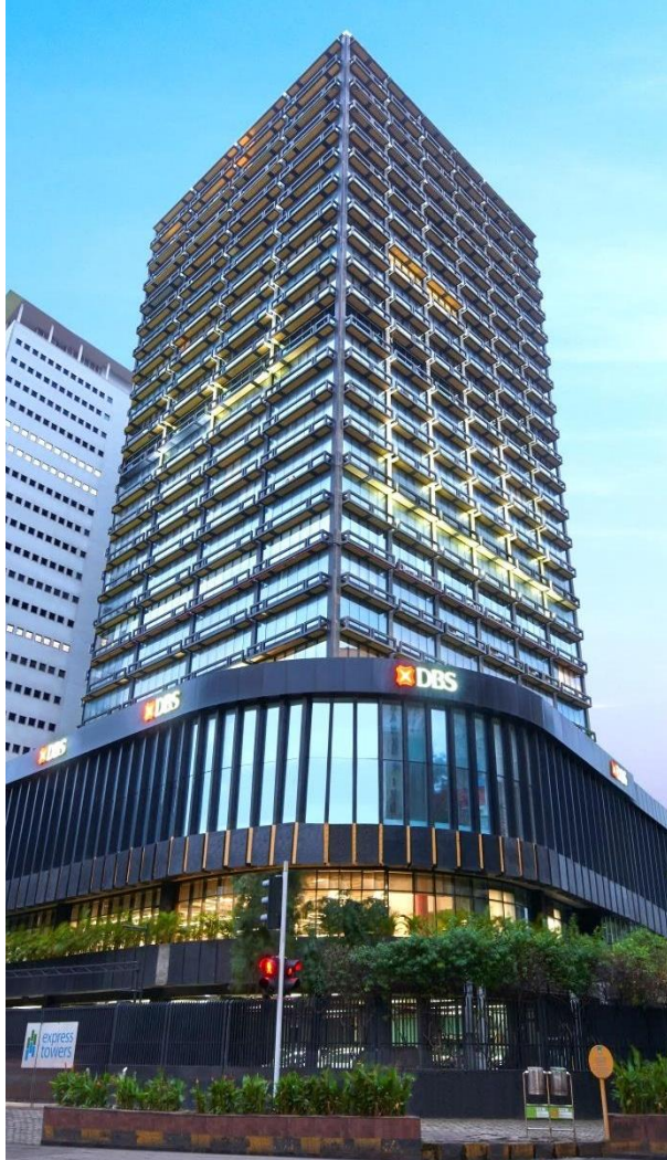
Express Towers Mumbai (0.5 msf)
