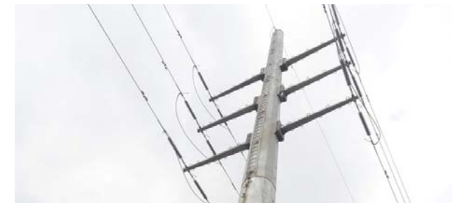
765 kV D/C - Tower
