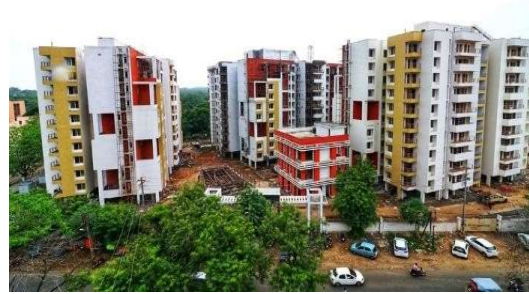
Construction of 222 Flats at Keelandev Tower, Bhopal for MP Housing & Infrastructure Development Board
