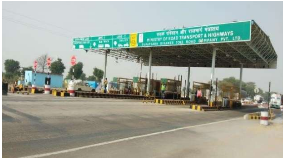
Development & Operation of Bikaner-Suratgarh Section of NH-62 (earlier NH-15) in the state of Rajasthan
