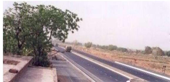
4 lane of km 41-51 of Agra Dholpur of NH-46 (earlier NH 3), in the state of Rajasthan
