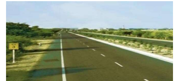
4 laning at Agra- Gwalior section, NH-2, in the State of Madhya Pradesh
