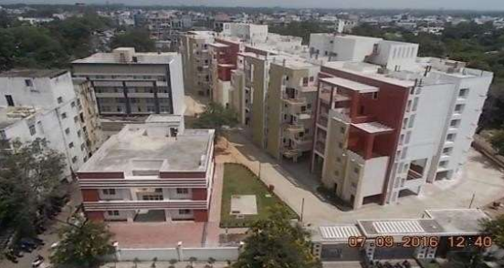
Construction of 92 flats at Mahadev Towers, Bhopal for MP Housing & Infrastructure Development Board
