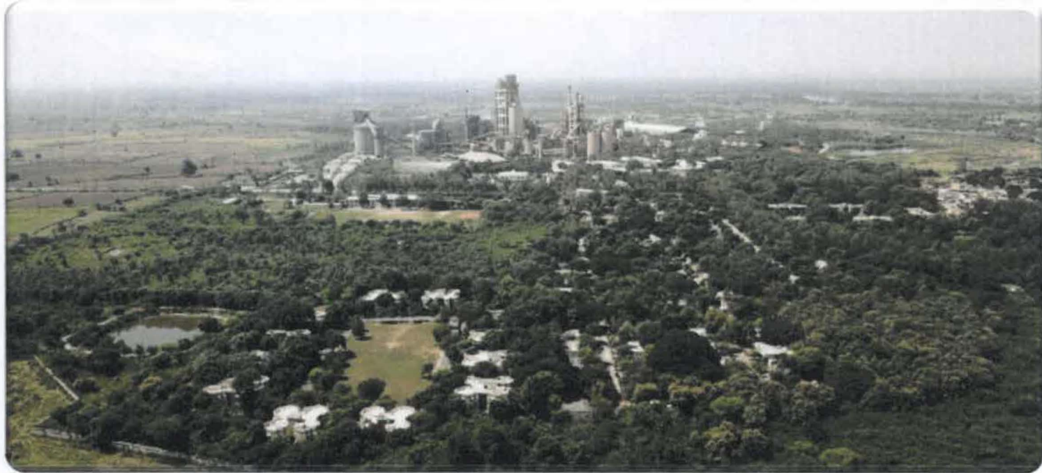
Bird's-eye view of clinker plant at Narsingarh, Damoh
