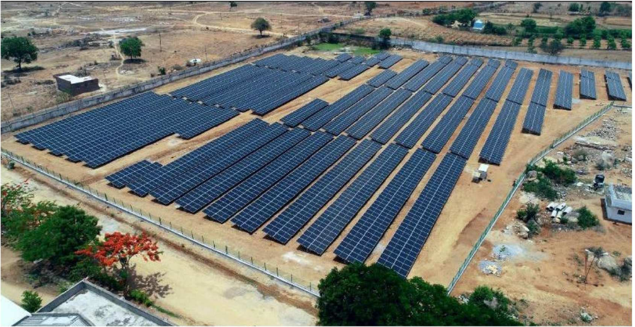
Solar power plant - Amanagallu
