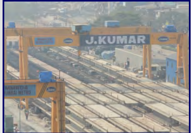
Girders for Elevated Metro
