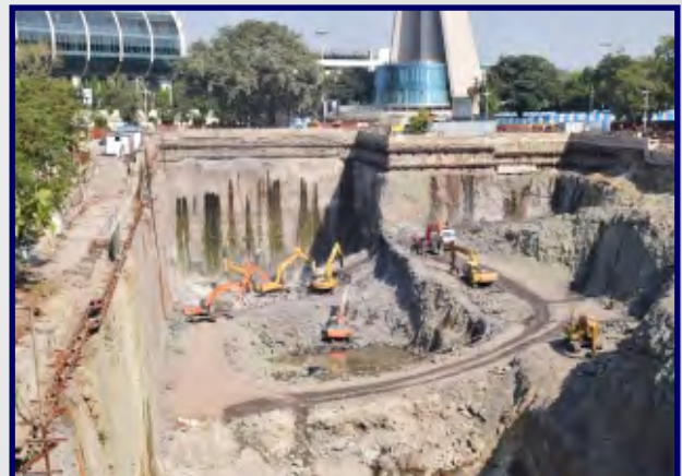
Domestic Airport Metro Station, Mumbai
