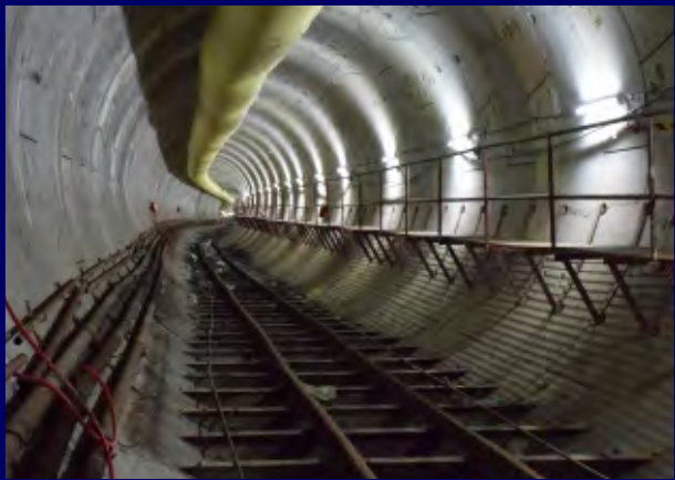
Tunnel From BKC to Vidyanagri
