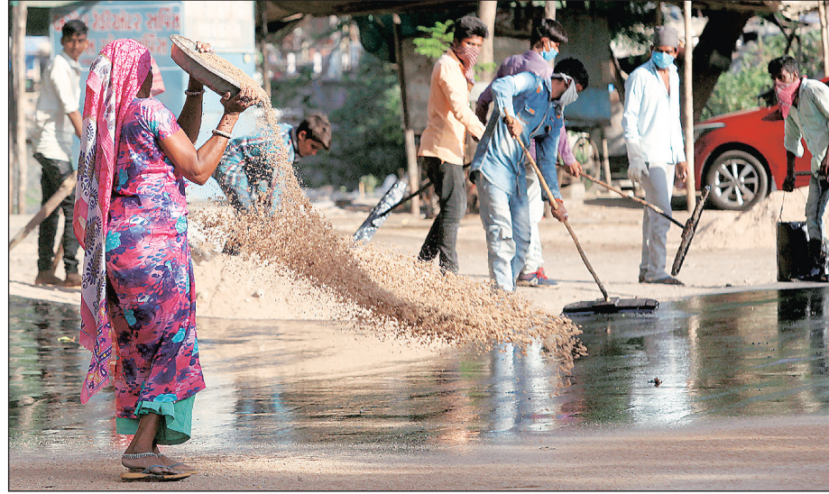
Road carpeting work under way in Vadodara on Tuesday. Bhupendra Rana
