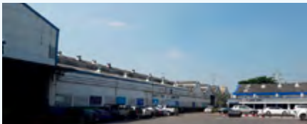
Usha Siam Steel Industries Public Company Limited [USSIL] – View of the plant situated at Pathumthani, Thailand
