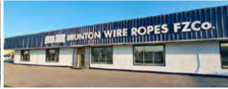
Brunton Wire Ropes FZCo (BWR) – View of plant situated at Jebel Ali Free Zone, Dubai
