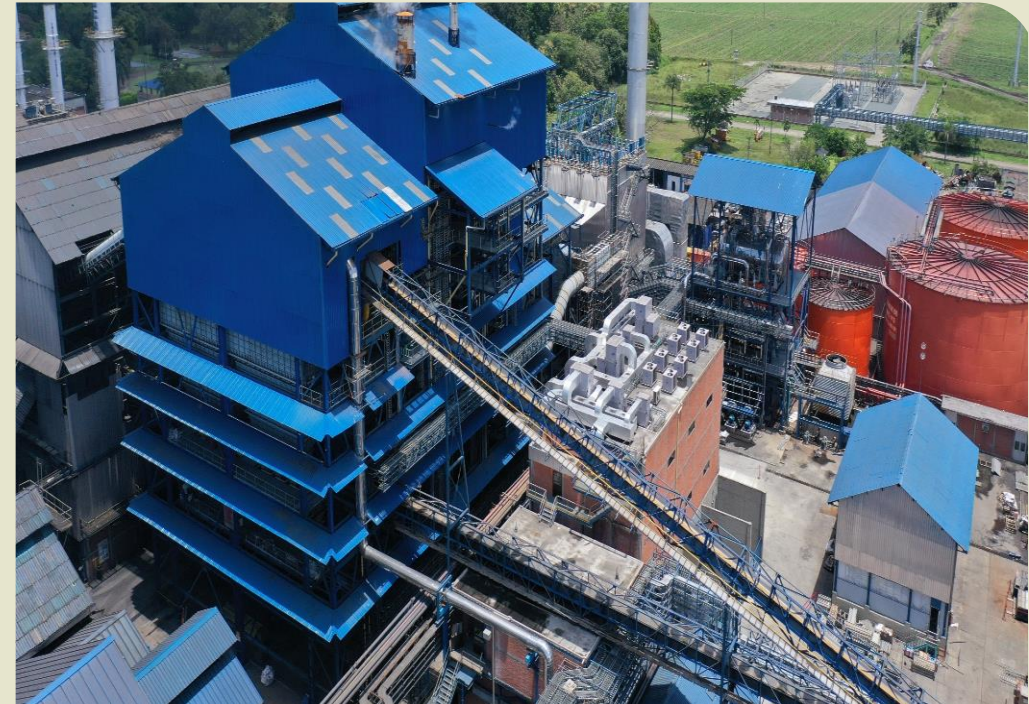
250 TPH Triple grate biomass fired boiler supplied in Latin America
