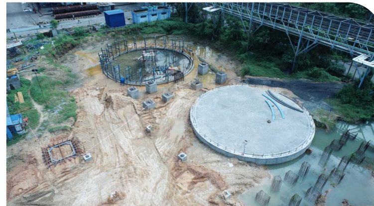
Multiple Site foundations ready for erection
