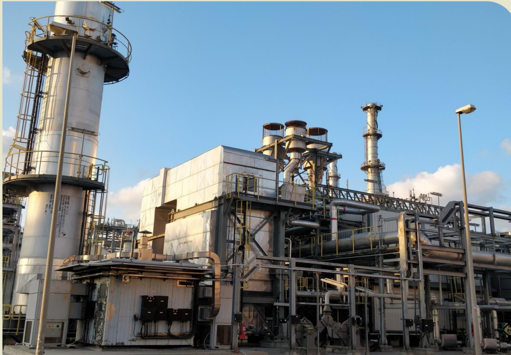
150 TPH gas fired boiler supplied to Egypt
