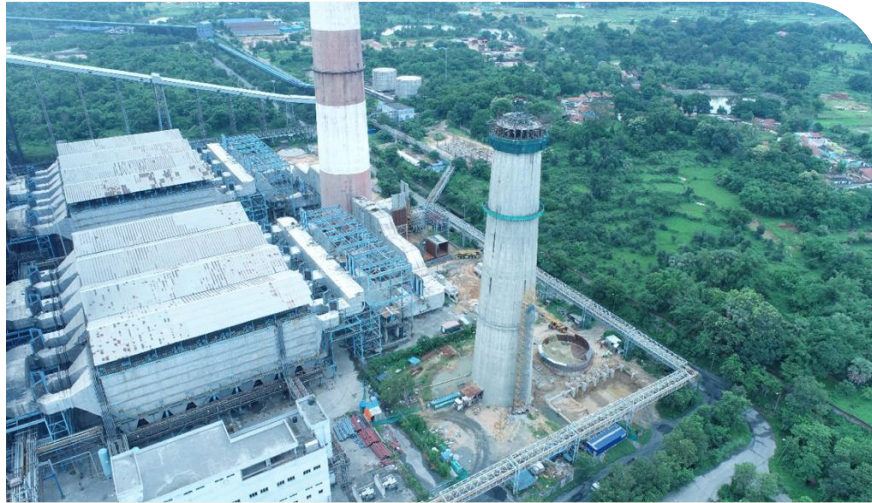
Wet Stack, Super Structure at 90 m
