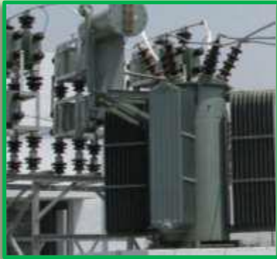
HT Passive Harmonic Filters
