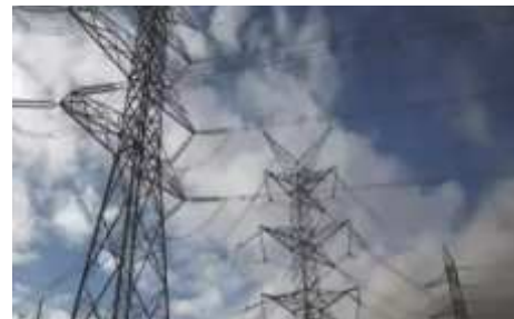
Noida Power Corporation Limited Project-Electification in Noida Products Used-Earthing electrodes & Steel Tubular Poles
