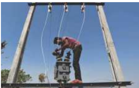
BSES Yamuna Power Limited Project-Earthing Electrodes Products Used-GI Pipes & Pole
