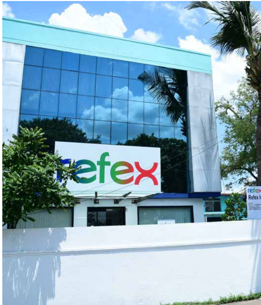
Refrigerant Re-filling Factory
