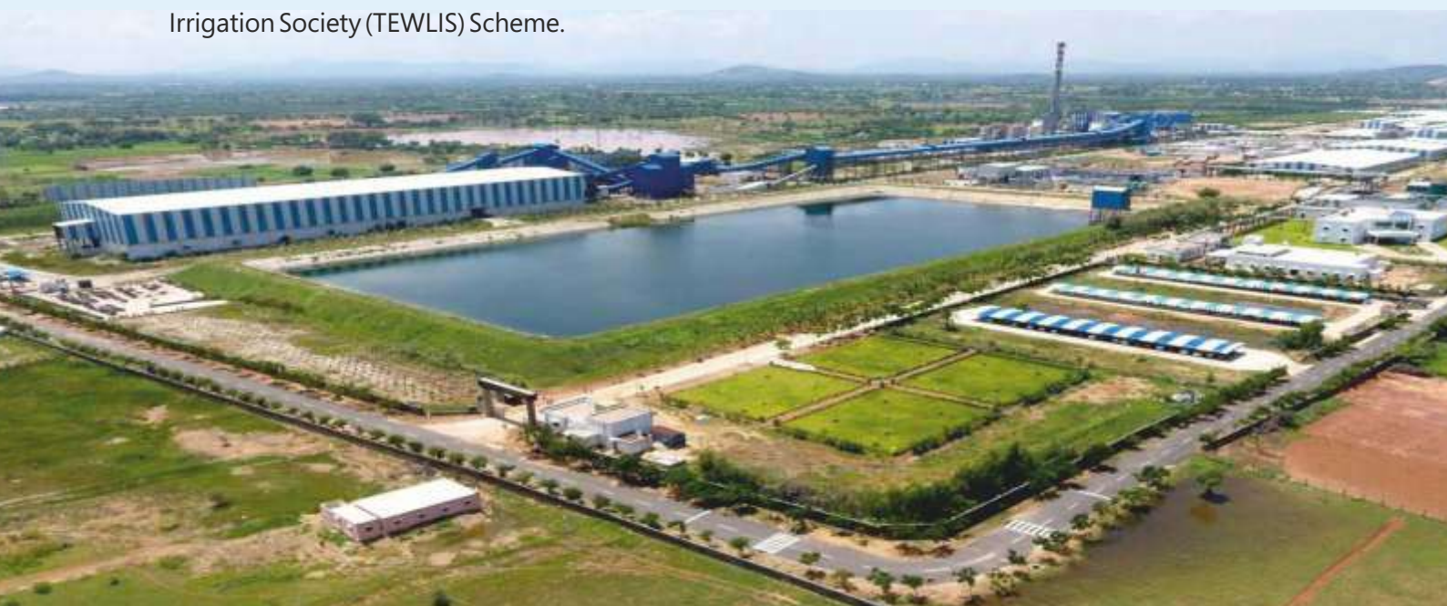
View of Water Reservoir at TNPL Unit II
