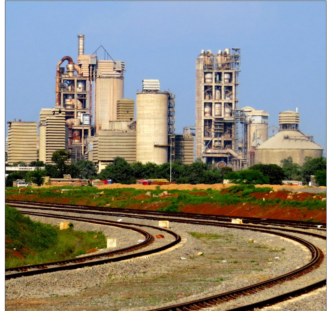
Sonadih Cement Plant
