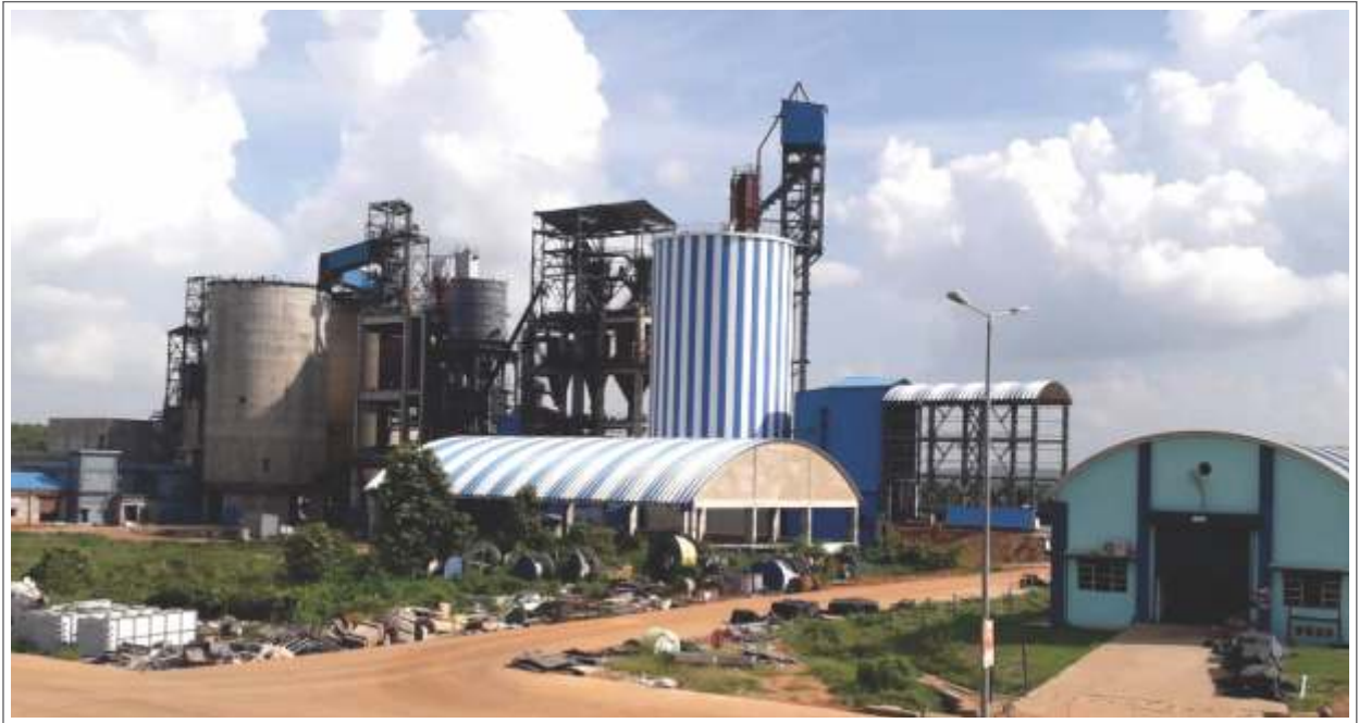
Cement Grinding Unit, Cuttack Odisha
