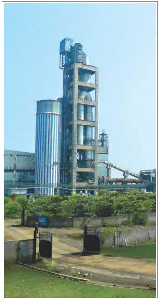
Integrated Cement Unit, Durg
