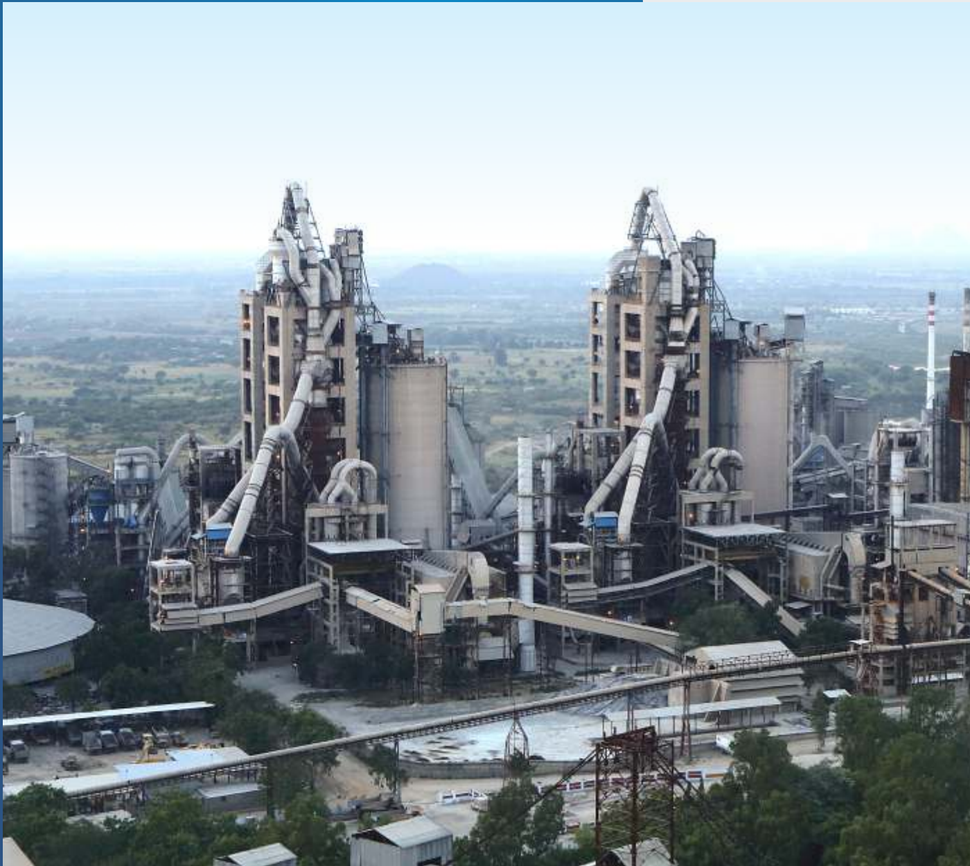
Integrated Cement Unit, Sirohi
