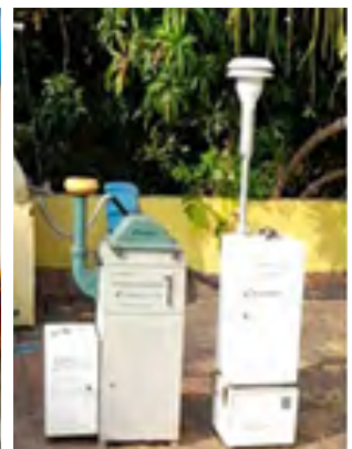
AAQ Station installed in Umangalam, Neyveli
