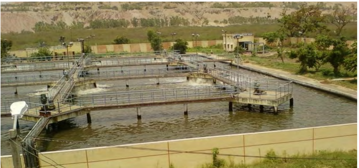
Municipal Sewage Treatment Plant – Neyveli Township
