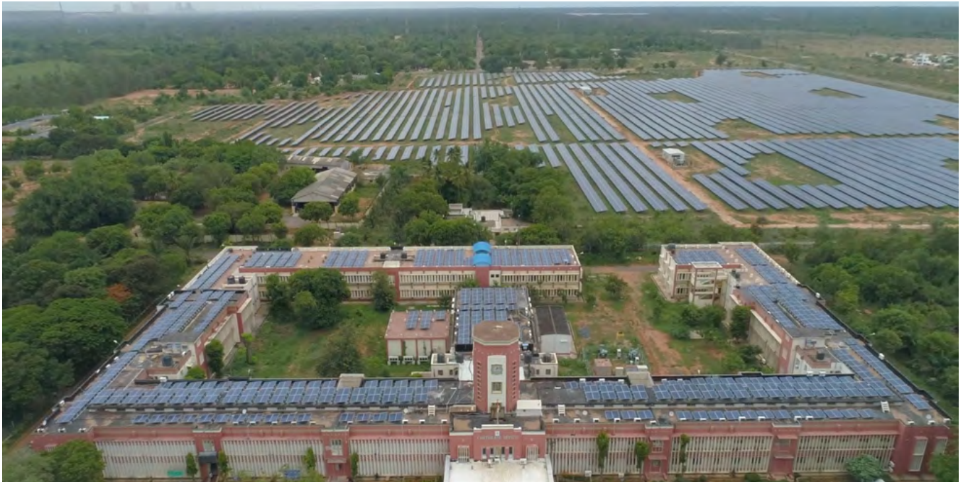
Rooftop Solar Plant at Corporate Office, Neyveli
