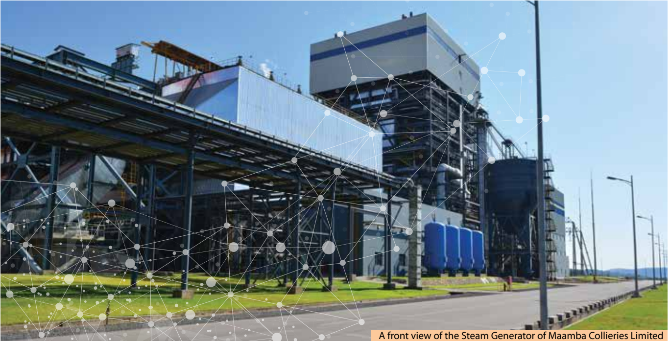
A front view of the Steam Generator of Maamba Collieries Limited
