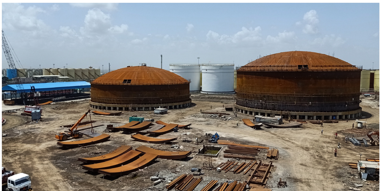
Kandla LPG Project Progress
