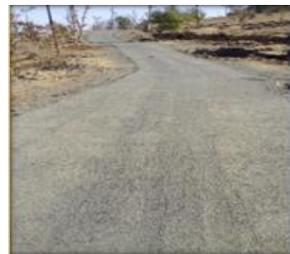
650 meter road constructed – 30 households connected (Zilla Parishad Cess Fund)
