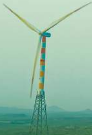
Nakhatrana Wind Farm, Gujarat, India
