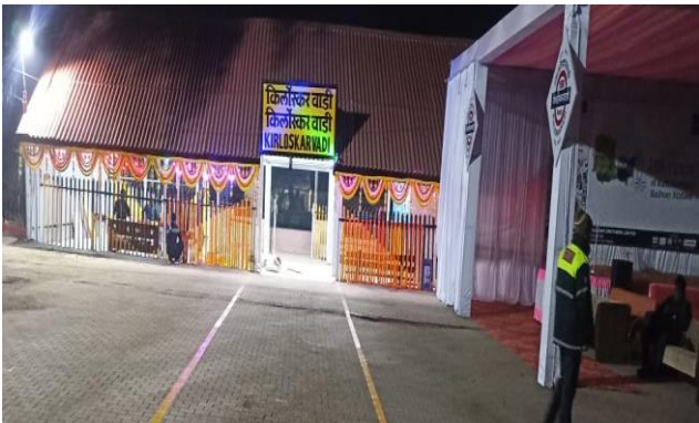
Renovation of Kirloskarvadi Station
