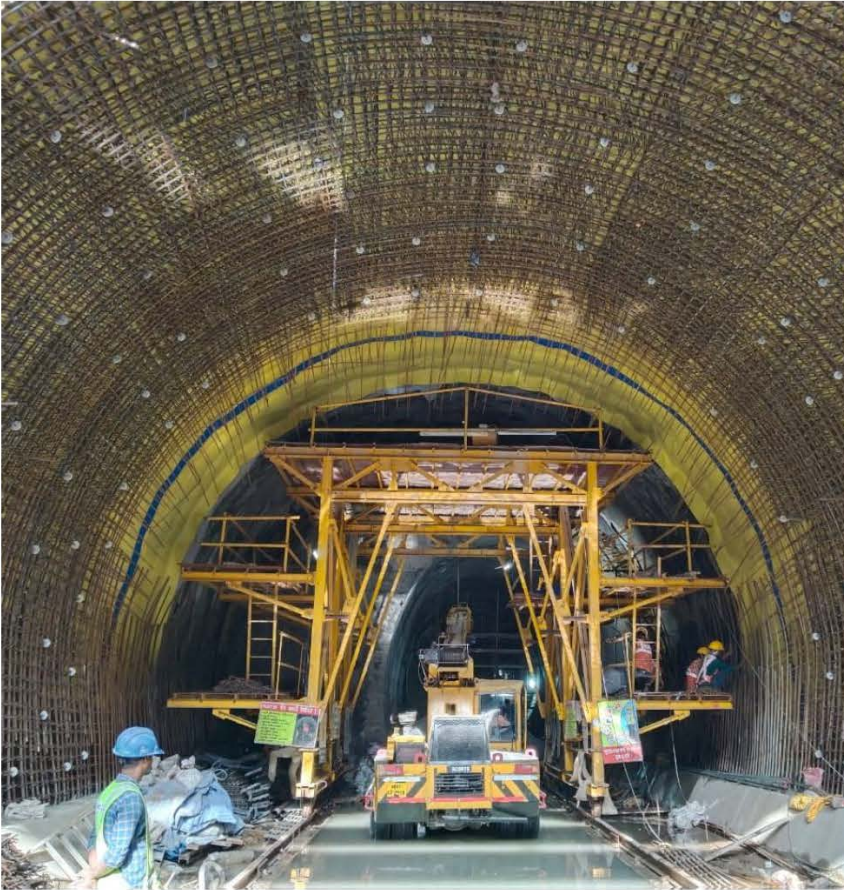
Girgaon Station: Civil work 59% complete.
