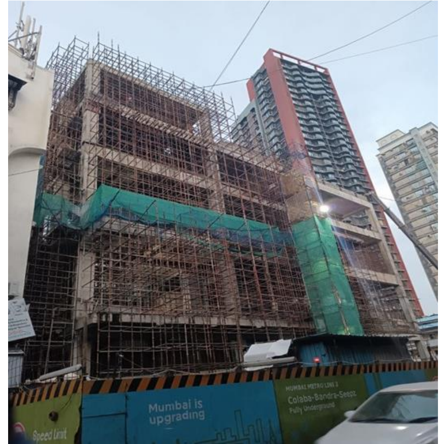
Kalbadevi Station: Civil works 80% complete. Finishing work in progress.
