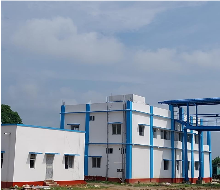
Toll Plaza Administrative Building
