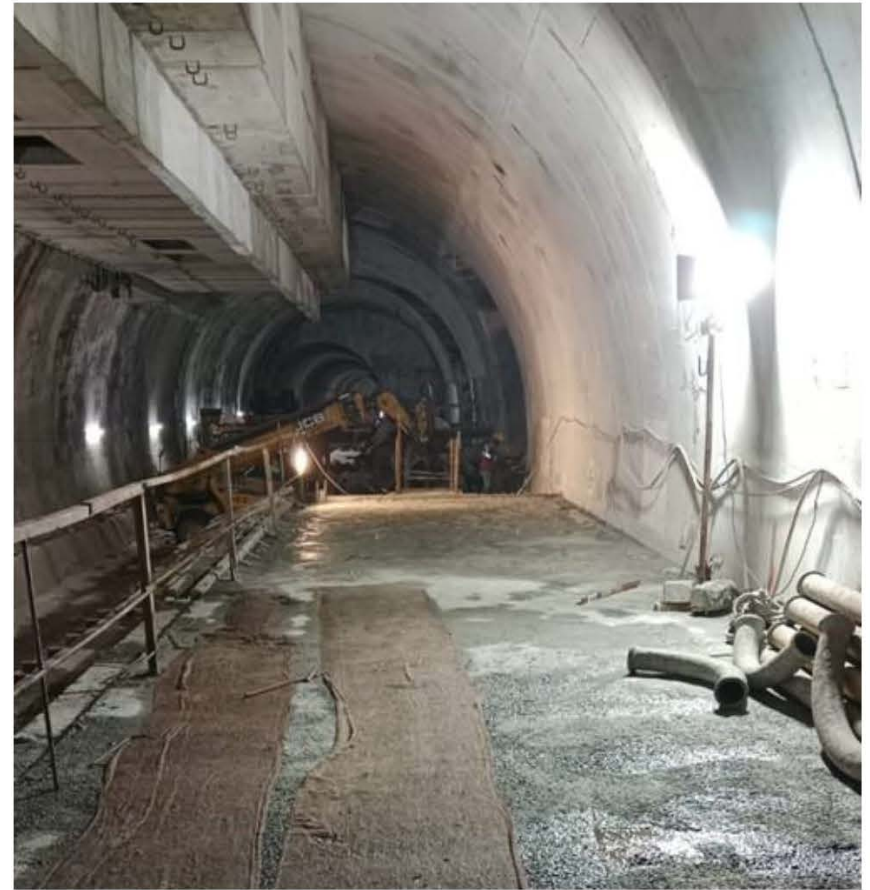
Grant Road Station: Civil Work 74% complete
