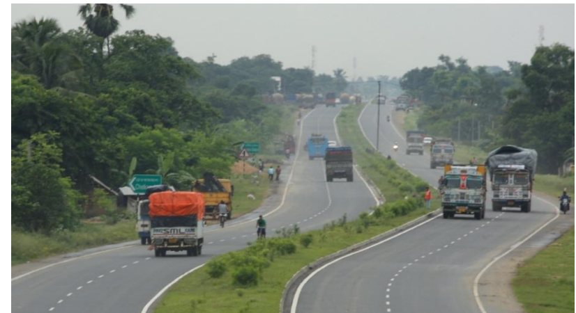
Km 341 (Farakka Raiganj Highway)
