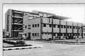
DAHEJ FACTORY Gujarat
