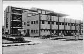
DAHEJ FACTORY Gujarat
