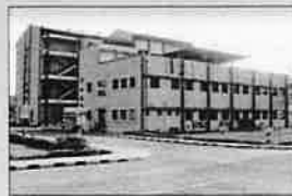
DAHEJ FACTORY Gujarat
