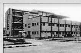
DAHEJ FACTORY Gujarat
