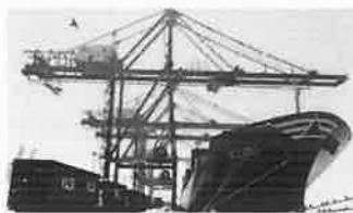
Shore power is a quicker and cheaper short-term solution that allows shipping companies to meet emission targets.
