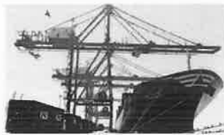
Shore power is a quicker and cheaper short-term solution that allows shipping companies to meet emission targets.
