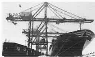
Shore power is a quicker and cheaper short-term solution that allows shipping companies to meet emission targets
