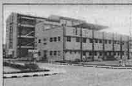
DAHEJ FACTORY Gujarat
