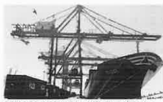
Shore power is a quicker and cheaper short-term solution that allows shipping companies to meet emission targets
