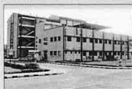
DAHEJ FACTORY Gujarat
