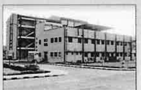
DAHEJ FACTORY Gujarat
