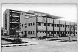
DAHEJ FACTORY Gujarat
