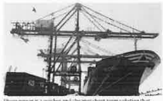
Shore power is a quicker and cheaper short-term solution that allows shipping companies to meet emission targets
