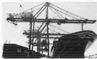
Shore power is a quicker and cheaper short-term solution that allows shipping companies to meet emission targets
