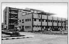
DAHEJ FACTORY Gujarat
