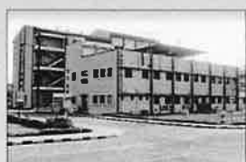
DAHEJ FACTORY Gujarat
