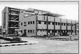
DAHEJ FACTORY Gujarat
