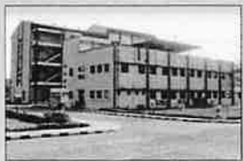
DAHEJ FACTORY Gujarat
