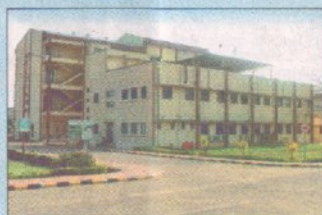
DAHEJ FACTORY Gujarat
