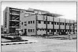
DAHEJ FACTORY Gujarat
