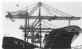
Shore power is a quicker and cheaper short-term solution that allows shipping companies to meet emission targets
