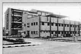
DAHEJ FACTORY Gujarat
