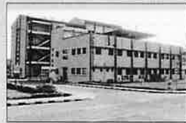
DAHEJ FACTORY Gujarat
