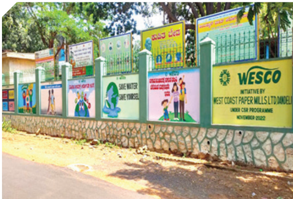
Compound Wall at Govt. Hospital - Dandeli
