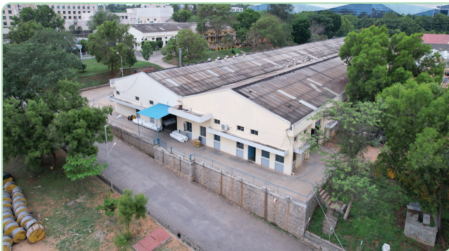
TELECOM CABLE DIVISION AT MYSURU
