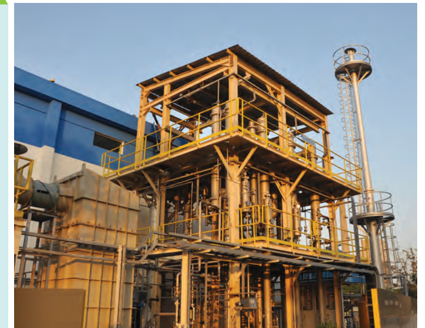
ZLD plant installation at the customer site
