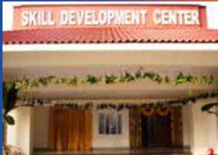
Skill Development Center at Antarvedipalem, East Godavari District, Andhra Pradesh
