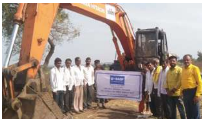
CSR intervention in partnership with NAAM Foundation in the area of water conservation by way of deepening and widening of existing water bodies in three villages of Hingoli district viz. Ambala, Bhingi and Waranga.
