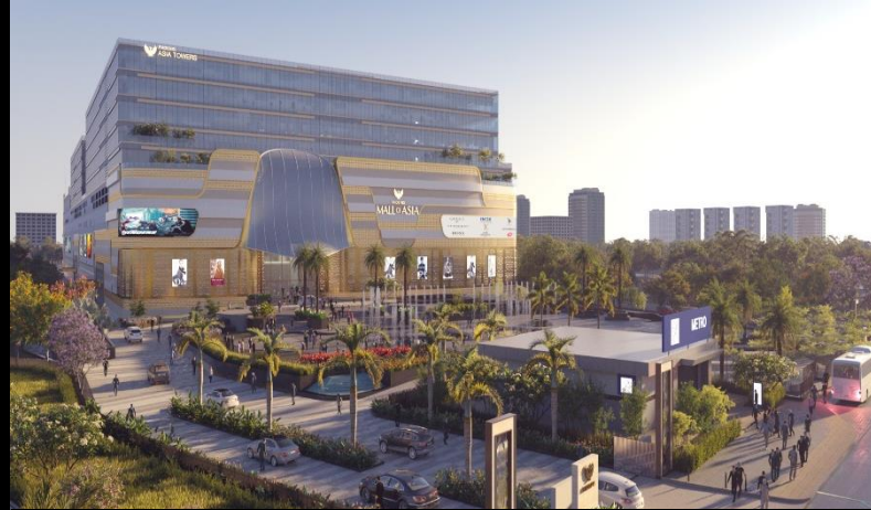
Upcoming Phoenix Mall of Asia + Asia Towers (Offices) Hebbal, Bangalore
